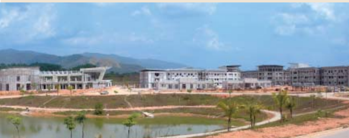
Panoramic view of the University of Nottingham Malaysia Campus under construction.
