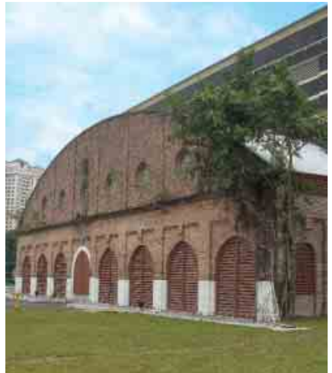
Use of UCO Supertex Woodgrain Planks at Kuala Lumpur Performing Arts Centre
