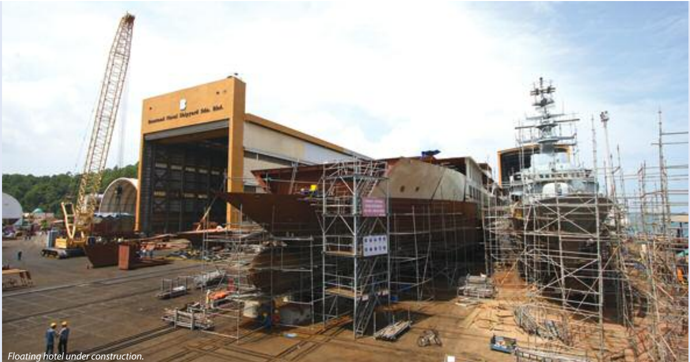
Floating hotel under construction.
