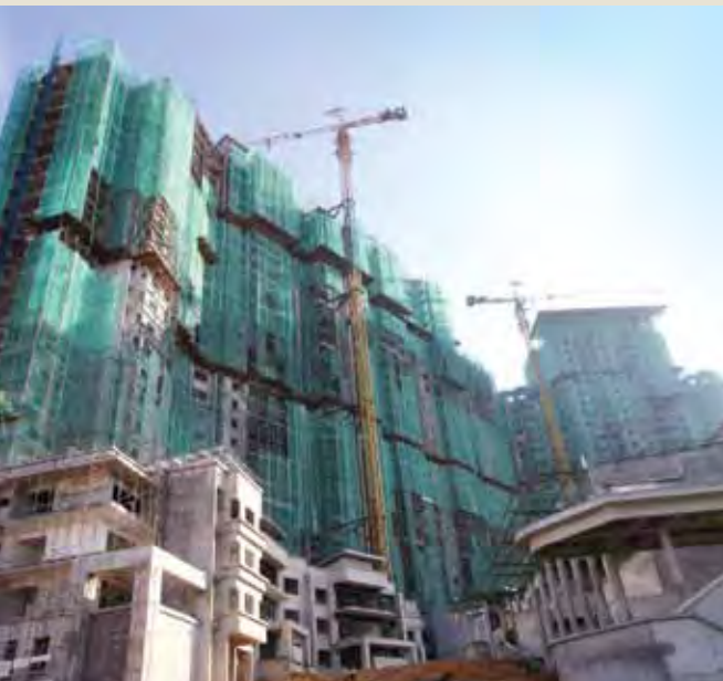
Surian Residences under construction
