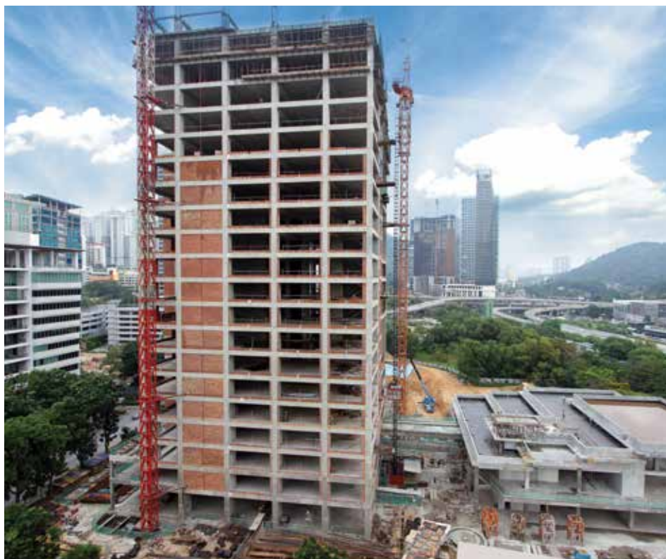
Nucleus Tower office building under construction
