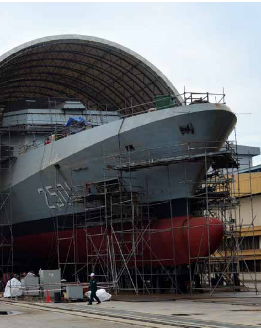
Ship repair and maintenance
